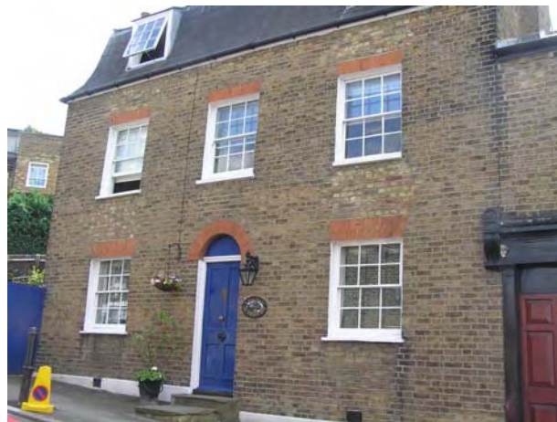
Picture 5.13 38 West Street, Harrow on the Hill
