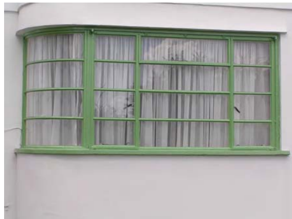
Picture 5.8 Original crittall window detail to Capel Gardens, Pinner View, Harrow
