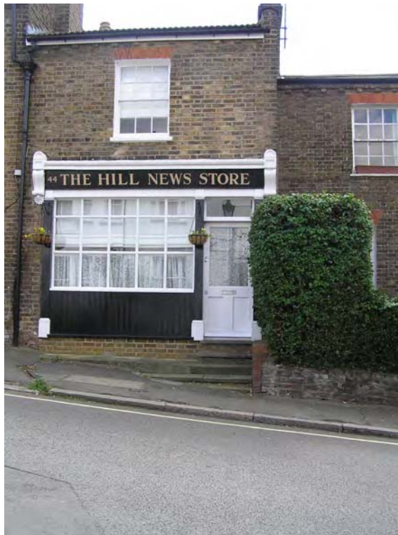
Picture 5.11 44 West Street, Harrow on the Hill
