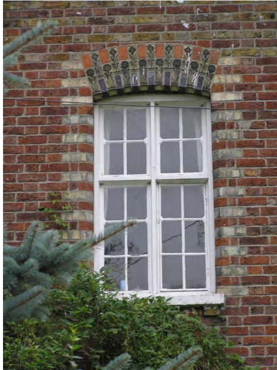
Picture 5.9 Original window detail to Pinnerwood Cottage, Woodhall Gate
